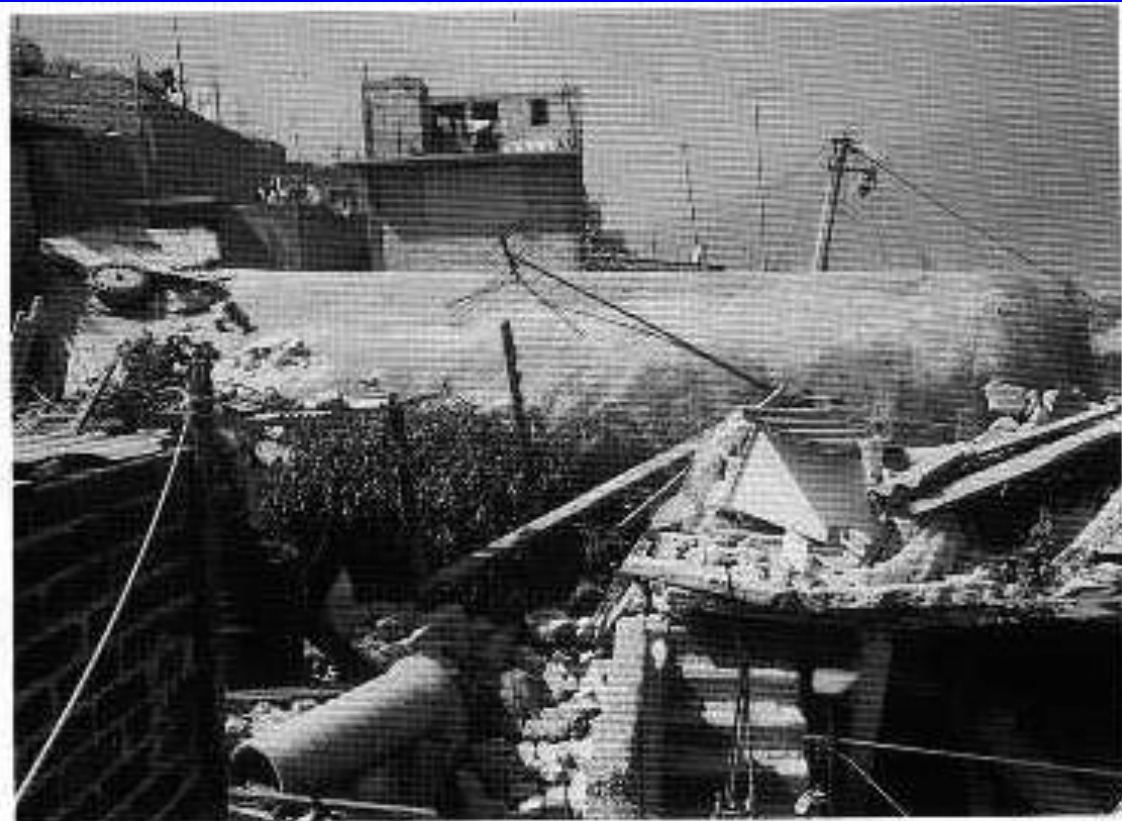
The cylindrical tank that flew furthest penetrated some 1,200 m into the housing area and crashed into a 2 storey house vacated one hour before.
