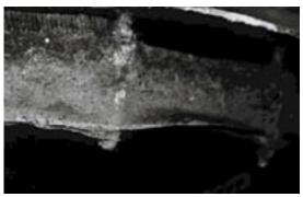
Fig 5.3 – Blocked filter on a floating roof drain cover.
