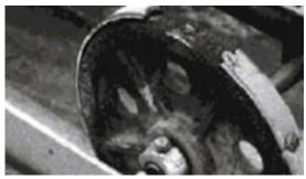
Fig 5.2 – Floating roof ladder wheel damaged – eventually the ladder will "jump" off the track and may tear the roof open.
