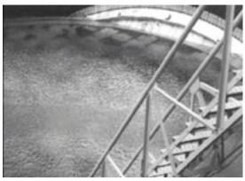
Fig 5.6 – Example of a sunken floating roof – caused by roof overloading
