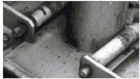
Fig 5.5 – Guide poles and the rollers can jam, causing roof jam and tilt
