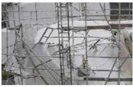
Fig 2.7 - Plastic sheeting used to cover the PV on the roof
