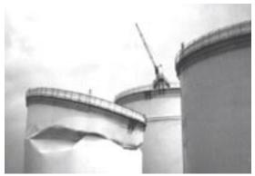
Fig 5.7 – Example of a tank collapse due to internal corrosion which was not detected properly.
