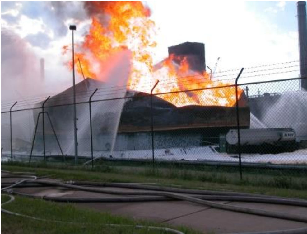
Figure 3 Photo from the Port Kembla fire in 2004. (Photo: Fire and Rescue NSW).
