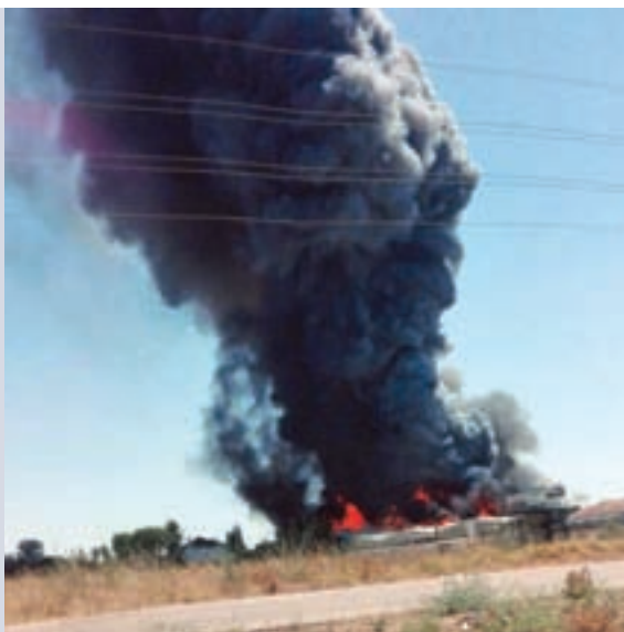
The dense black smoke generated by the burning olive oil prevented firefighters from entering the buildings. (Images: @Rafaruiz76)
