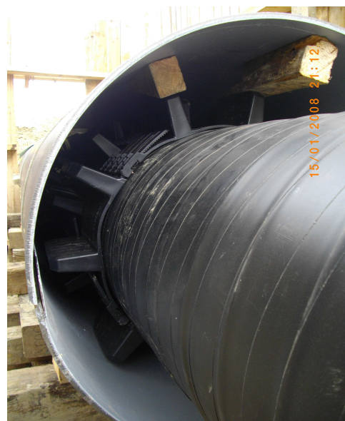
Copyright: Pipeline operator
