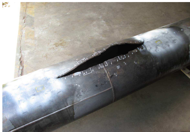
Copyright: Pipeline operator
