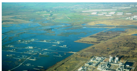
Figure 5 : SABIC Brinefields and the flood defence breach, source Environment Agency
