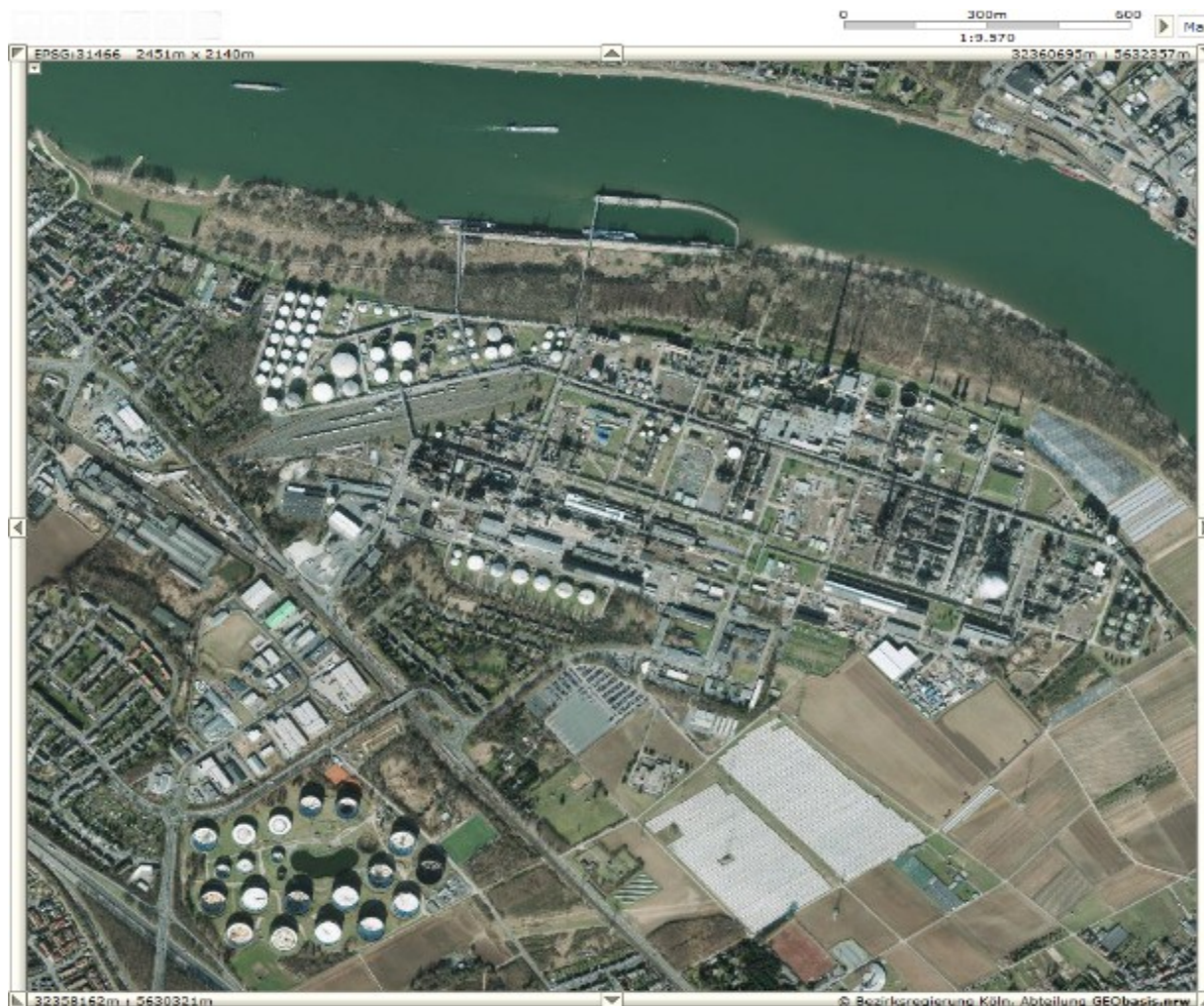
Figure 1: The Refinery south of Cologne is connected to the tank field (down left) by sub-surface pipelines
