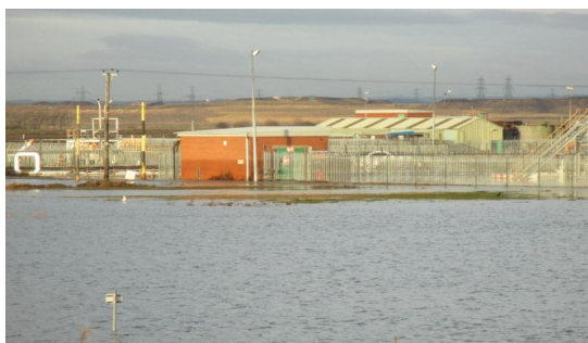
Figure 6 : Control room on the Brinefield – note flood level mark on control room wall, Source Sabic UK Ltd
