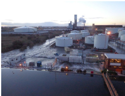
Figure 2 - View of terminal being flooded from ship moored up on jetty, source Cleveland EPU
