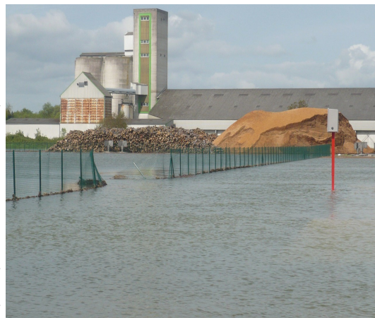
Wood storage at the plant overwhelmed by water (Source: DREAL Champagne-Ardenne)
