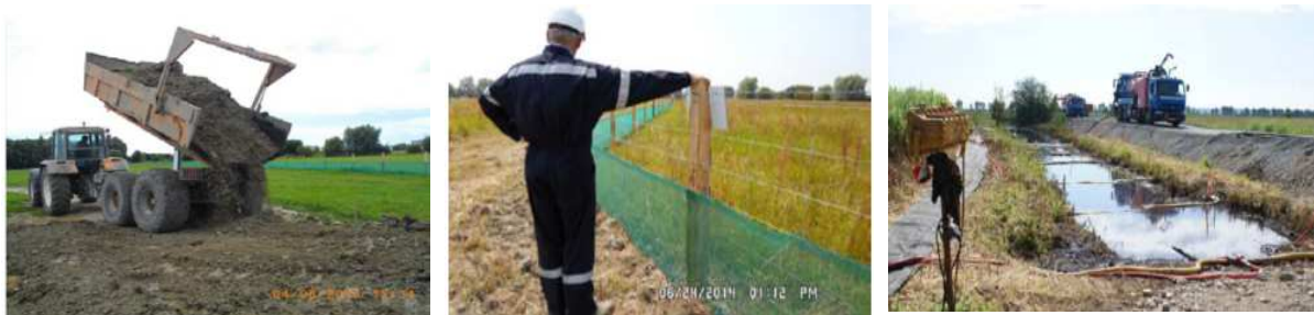
Copyright: Pipeline operator
