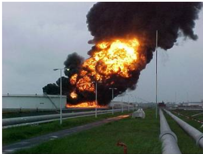
Nigeria 2002 – Note crude flowing outside bund
