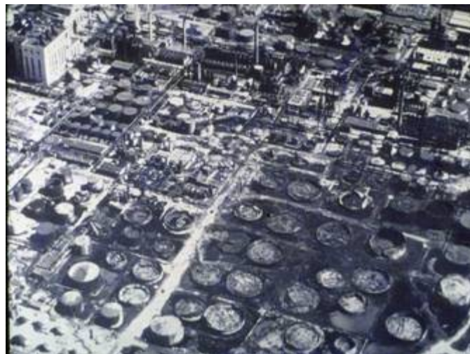
Whiting Oil, 1955 damage caused by domino effects of repeated boilovers
