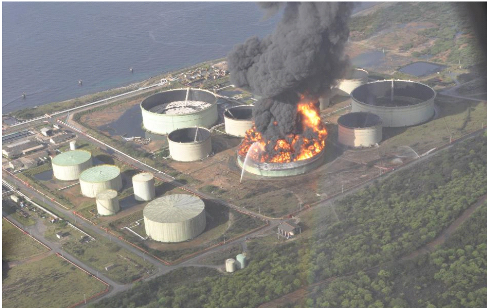
Figure 4 Photo impression of a later stage of the fire in the naphtha tank, including some fire fighting activities.
