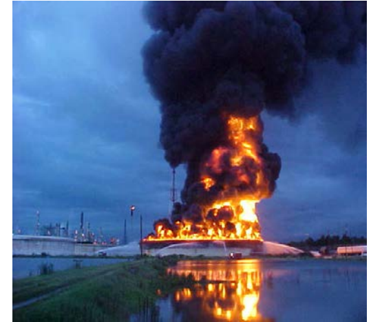
Crude Oil Tank Fire
