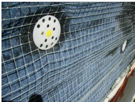
Figure 1.4 Mechanical fix of aerogel blankets in external insulation (Aspen Aerogels 2012).
