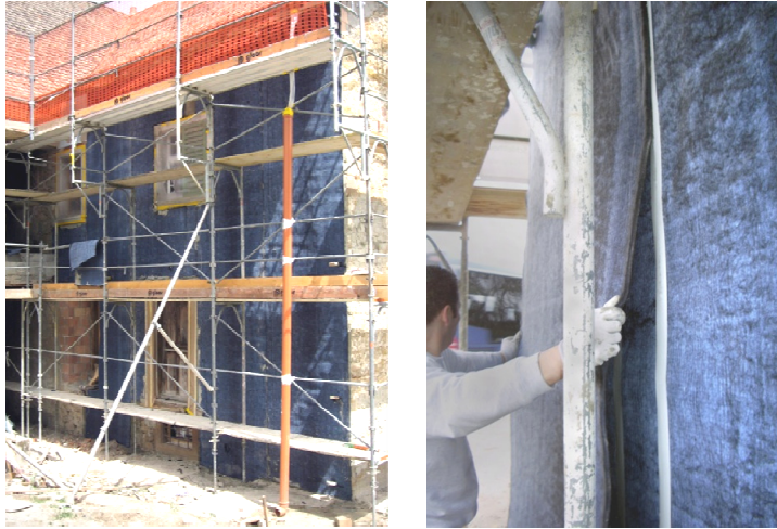
Figure 1.3 External insulation (Aspen Aerogels 2012).
