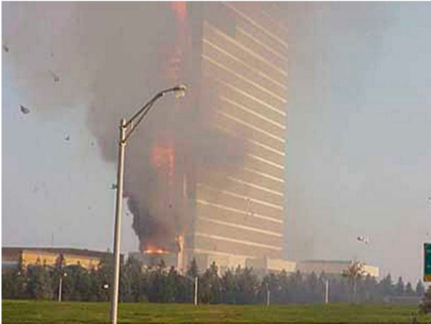
Fig. 86.23 Fire at the water club tower (Courtesy of J. Foley, Atlantic City Fire Department)
