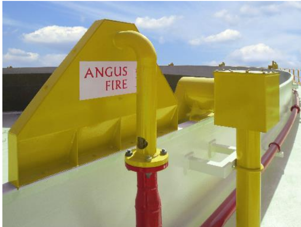
Rimseal pourer (left), full surface pourer (right)
