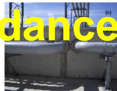
Above - Fig 2.3.2.1(e). Pictures (a) and (b) showing bund sealing (note impermeable membrane). Pictures (c) and (d) show good practice sealing of bund transits and poor practice with no seals. NB: Sealant materials should be sufficient to withstand fire conditions.
