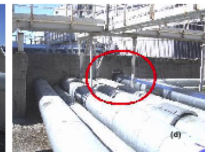
Above - Fig 2.3.2.1(e). Pictures (a) and (b) showing bund sealing (note impermeable membrane). Pictures (c) and (d) show good practice sealing of bund transits and poor practice with no seals. NB: Sealant materials should be sufficient to withstand fire conditions.
