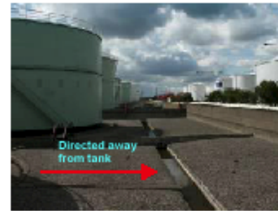
Above - Fig 2.3.2.1(c). Spill channels should lead away from tanks and preferably be fitted with flame traps to prevent fire spread
