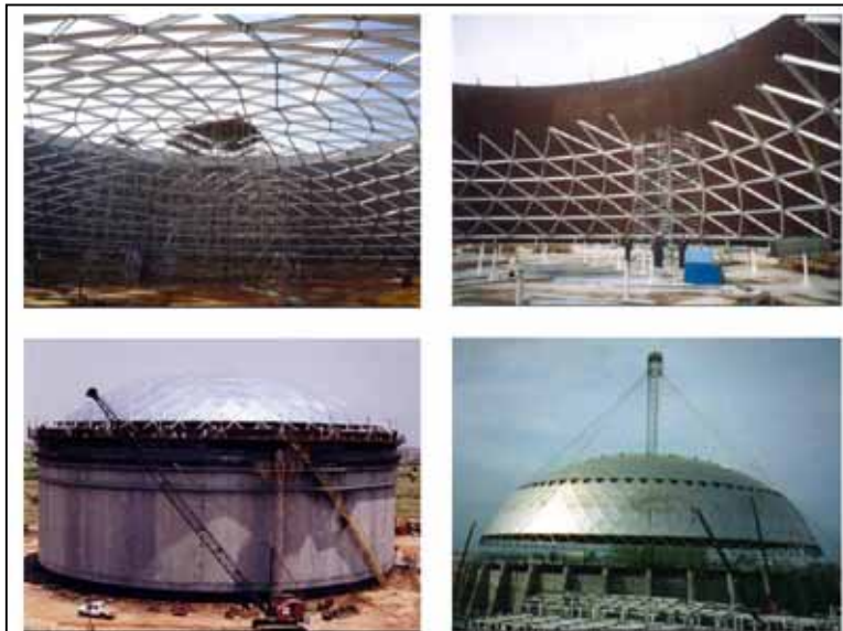
Figure 2.2.1 - Geodesic domes can be built on the ground and lifted into place or built directly on the existing floating roof tank and winched into place. A variety of methods are available for erection, including "jack stand" erection (top), "grip hoist assembly" (bottom left) and "tower assembly" (bottom right).
