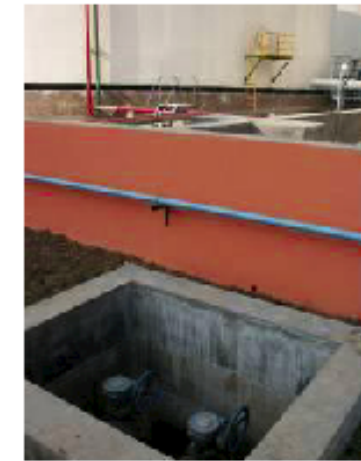
Above - Fig 2.3.2.1(c). Spill channels should lead away from tanks and preferably be fitted with flame traps to prevent fire spread
