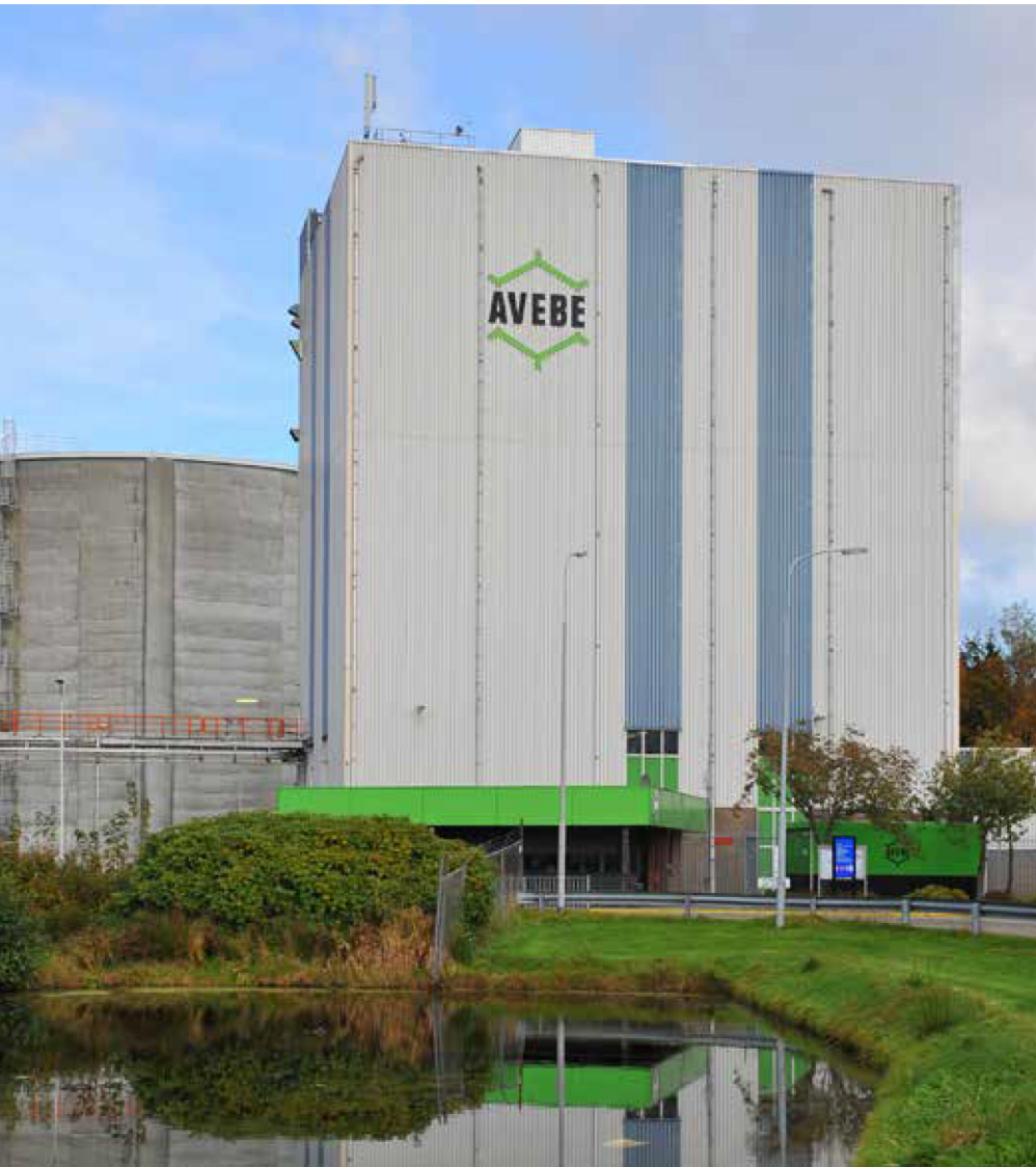
◀ AVEBE Foxhol, industrial unit for processing and storage potato starch.
